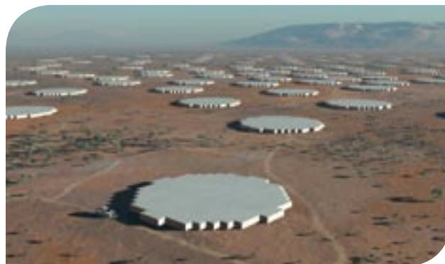
Dense Aperture Array. © Copyright SKA: enquiries@skatelescope.org
